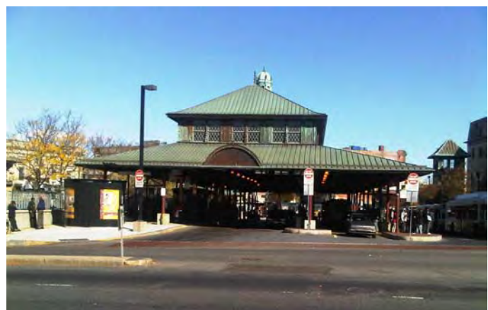
Dudley Station is a transportation hub when 16 major bus lines converge.
